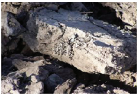
Fig. 4. Break up of compacted clay with a ripper.
